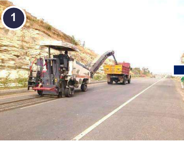
Milling & Profile Correction
