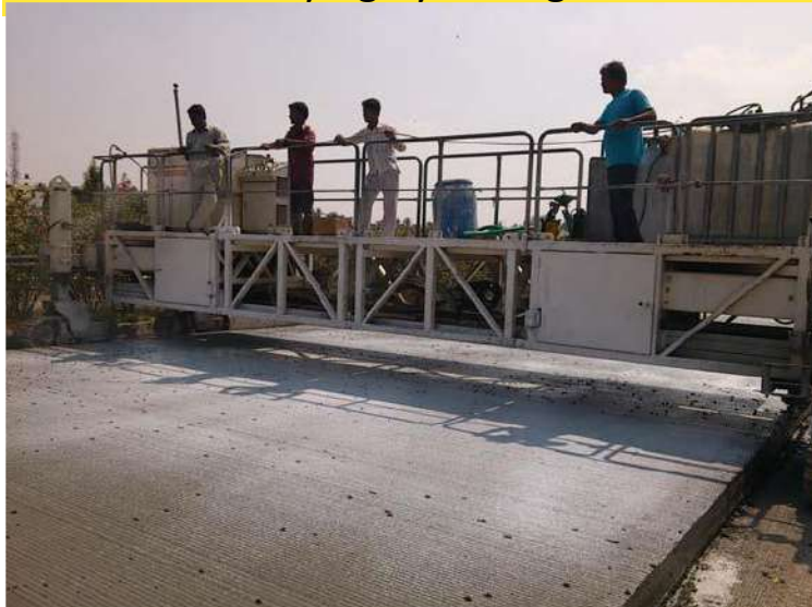
Curing Compound Spraying
