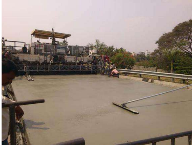
Surface Finish by Bull Float
